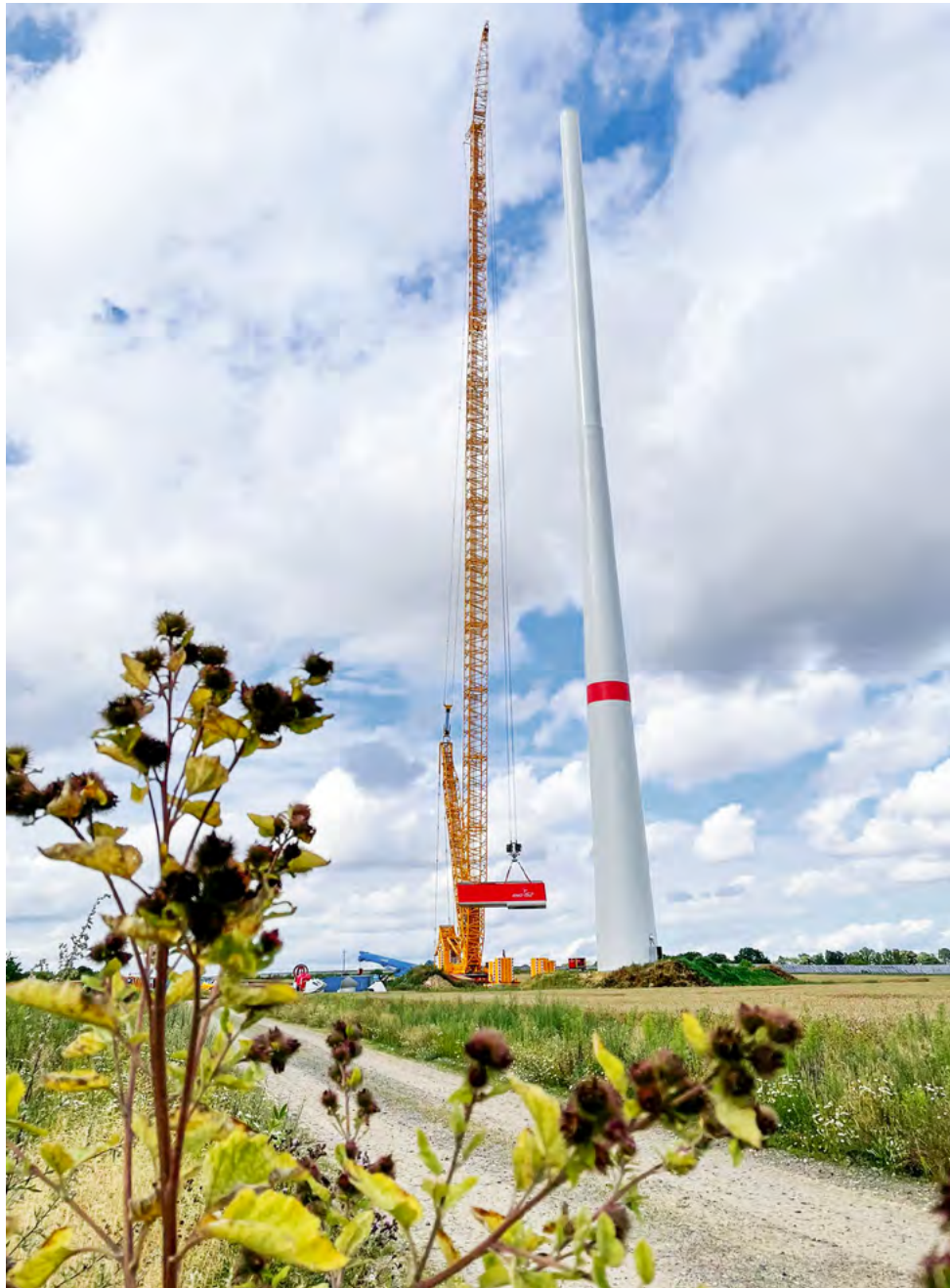
The hub is lifted onto the pivot, where it is completed and installed.
